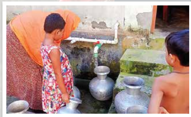
Desalination Plant at Khejurtola Govt Primary Hospital under Barguna District
